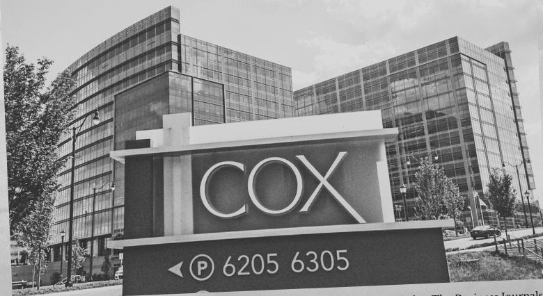
Cox Headquarters in Atlanta, GA
